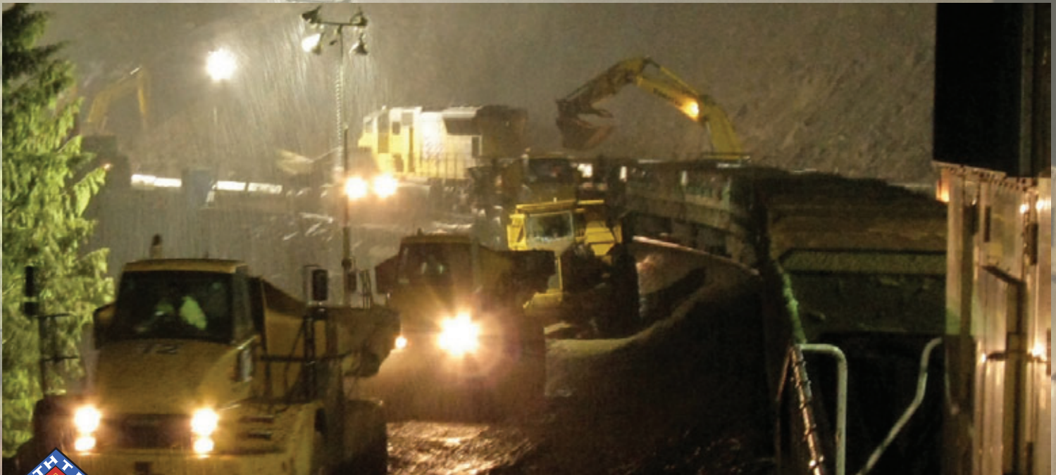
Night operations on the Frazier Slide
